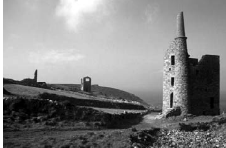
1: Pumping engine house at West Wheal Owles mine, © Adam Sharpe, Cornwall County Council
